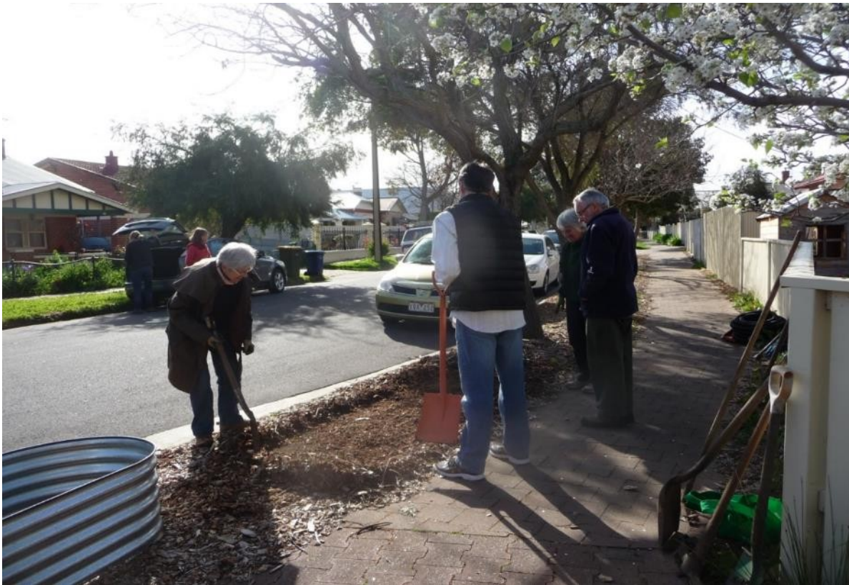
Installing a verge bed at Black Forest – Christy Spiers' place. Russ always pitched in.
