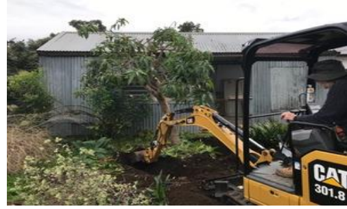
4.1. the excavator digging the tree out.
