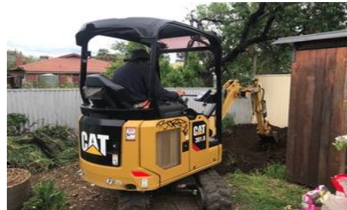
5. excavator delivering it to its new spot
