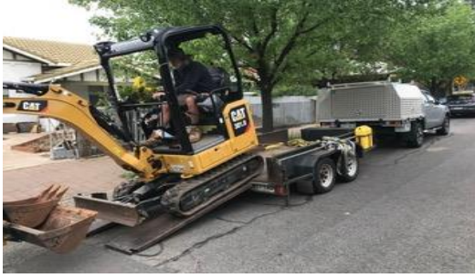
3. the arrival of the excavator
